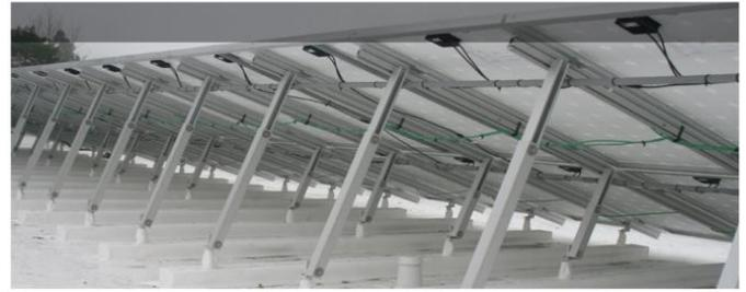
**Figure 2:** Anchored PV array on rooftop
